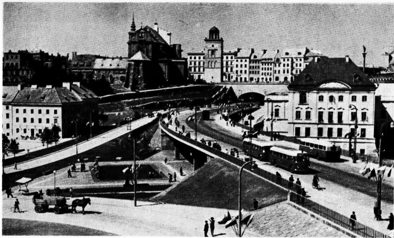
PLATE 2. The eastern entrance to the tunnel under the Old Town on the new east-west highway (page 30).
